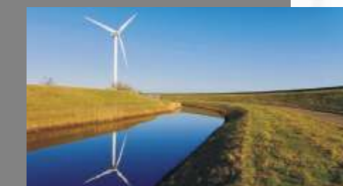
Strengthening the stability of dams and embankments
